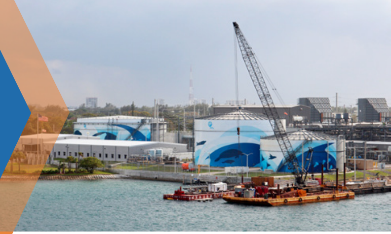
Florida Power & Light storage tanks sit along Manatee Lagoon in West Palm Beach at this natural gas plant. Photo taken May 2018.
