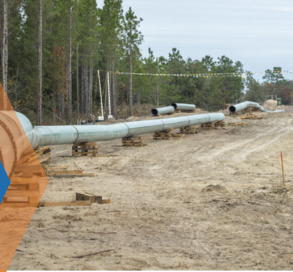
New natural gas pipelines being installed in Gilchrist County.
