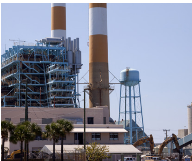
This Florida Power & Light power plant in Riviera Beach was demolished in 2011 and replaced with a natural gas plant.
