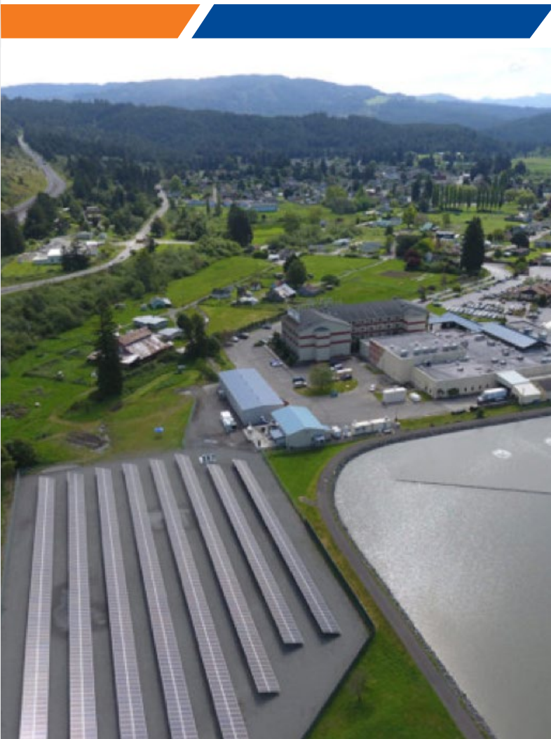
Blue Lake Rancheria. Source: Schatz Energy Center
